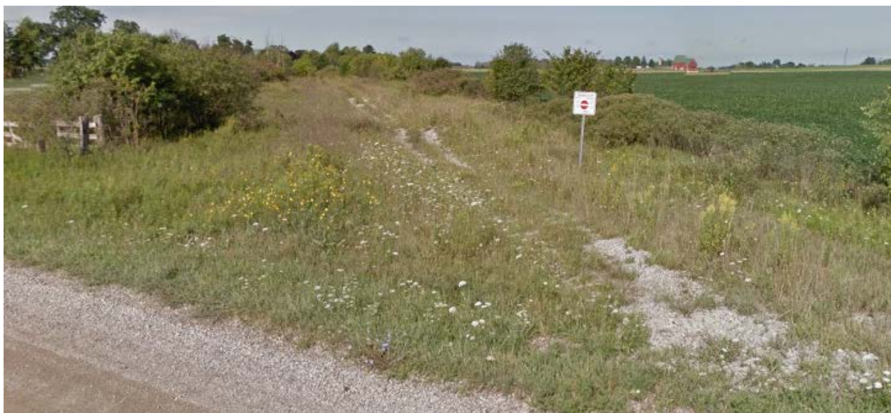
Figure 1-1: View of the Eastern Boundary of the Project from Stafford Line, Facing West. Google Street View Image Taken in August 2016
